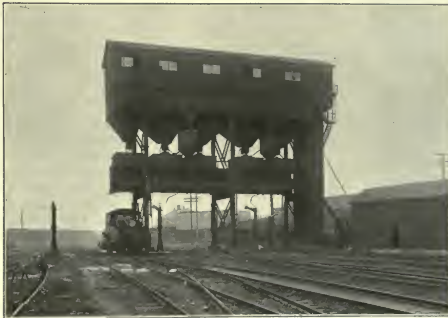
FIG. 668. FACILITIES TO BE ABANDONED. Mechanical coaling station of the Lake Shore & Michigan Southern Railway at 63d Street and Michigan Avenue. This station has a storage capacity of 600 tons. In the event of electrification, this station will be rendered worthless to the railroad in its present location.
